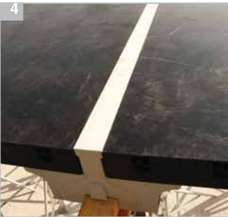
Block the panels onto the Y-beams
