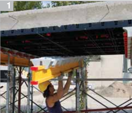
Remove the H-beams
