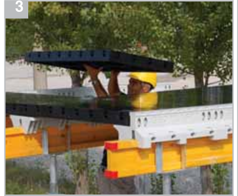
Place the GEOPANEL® 120 panel
