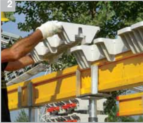
Place the H-beam
