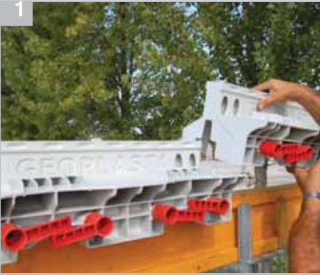
Place pre-assembled Y-beam and wedges
