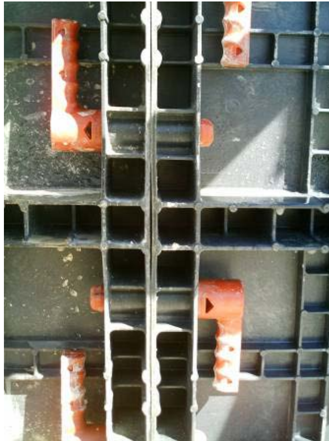
Photo 8: view of a gap opened between two panel elements, again with slight fluid percolation.
