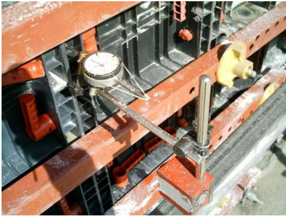
Photo 5: view of a positioned, numbered, and calibrated deflectometers.
