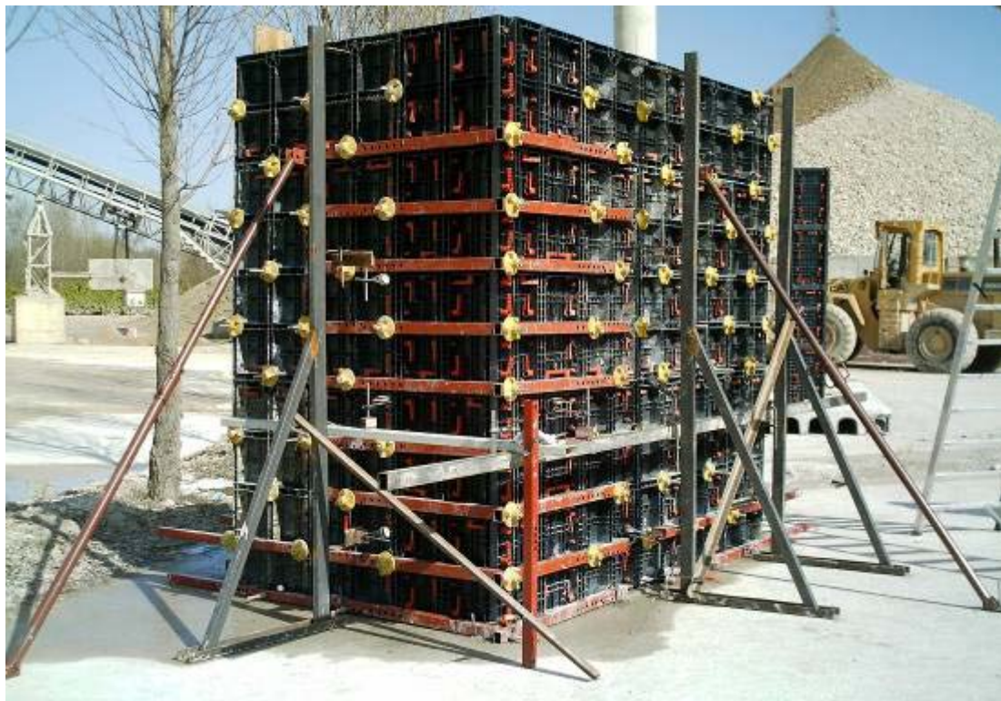
Photo 4: view of southern and western sides, with all the deflectometers already positioned, numbered and calibrated.
