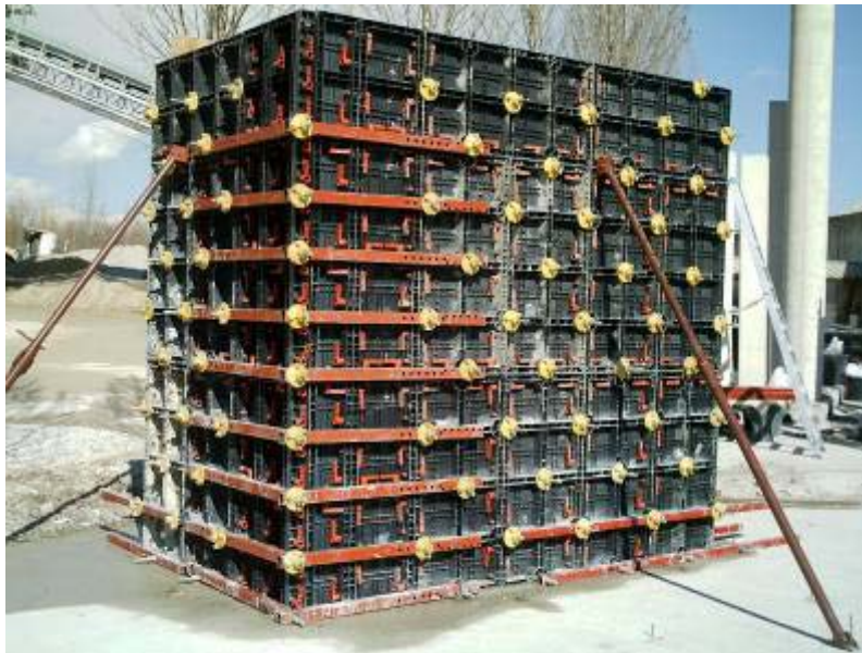
Photo 1: external view of the test form (the short edge faces west, the long edge faces south)
