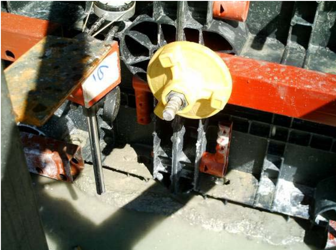
Photo 6: shown from the west side at the end of the test; some slight percolation of the concrete is visible through the gaps in the form panels and onto the ground.
